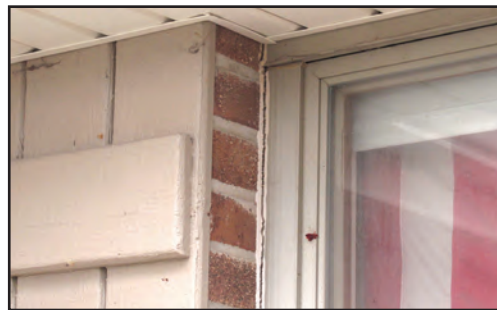
Sealant deterioration
