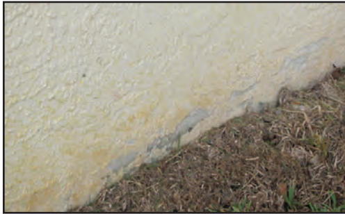
Finish deterioration
